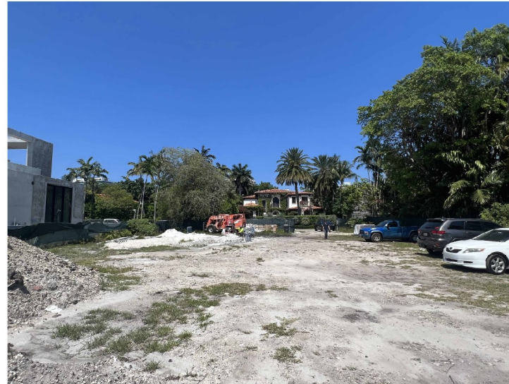
SITE VIEWS LOOKING EAST - STREET SIDE
